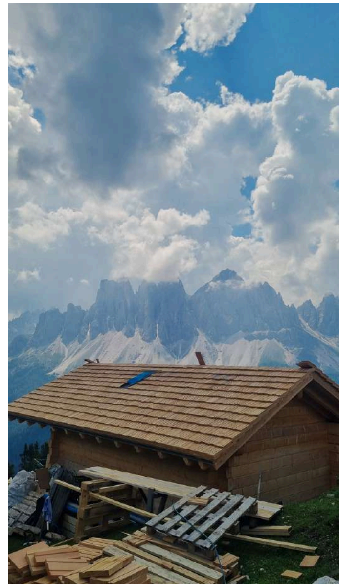
The cold shell for the new hut.
